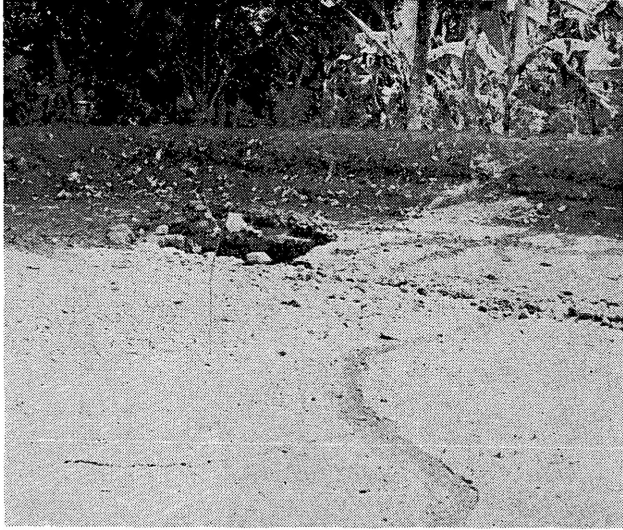
Photo 3. Sump to facilitate fish removal dug off-center in a minapadi ; Sukabumi, Indonesia.
