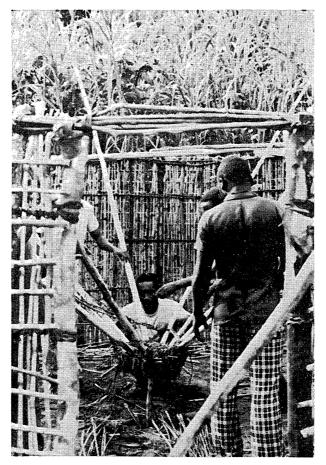
Photo. 3. The lower ends of the rafters rest on the upper edge of the wall-frame.
