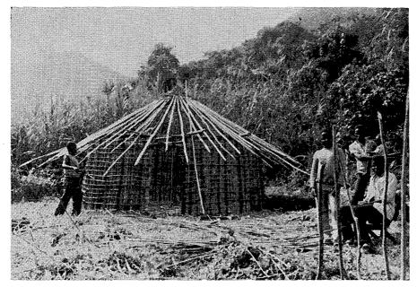
Photo. 4. The roof-frame is turned over and erected properly on top of the wall frame.
