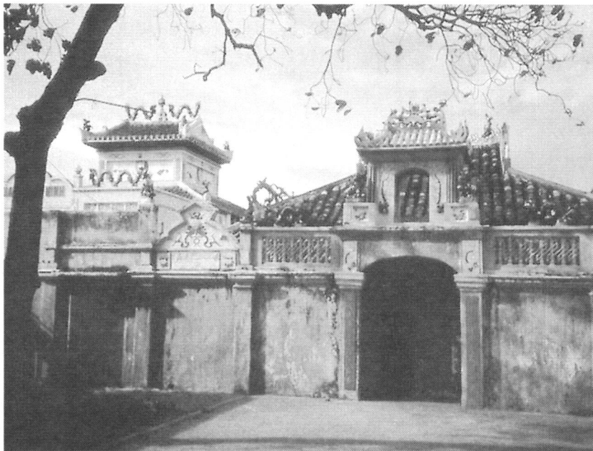
Photo 1 The shrine building at Van Thuy Tu, Phan Thiet
