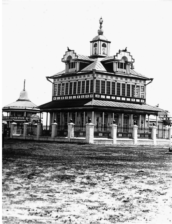
Photo 8 The Kalmyk Buddhist Temple near Volga. The beginning of the 20 th century
