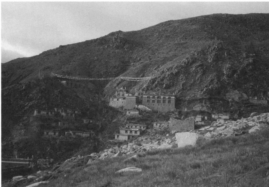
(1) sMan ri Monastery, Plate 2 sMan ri, ruins and new buildings (Photo Dondrup Lhagyal 1996)
