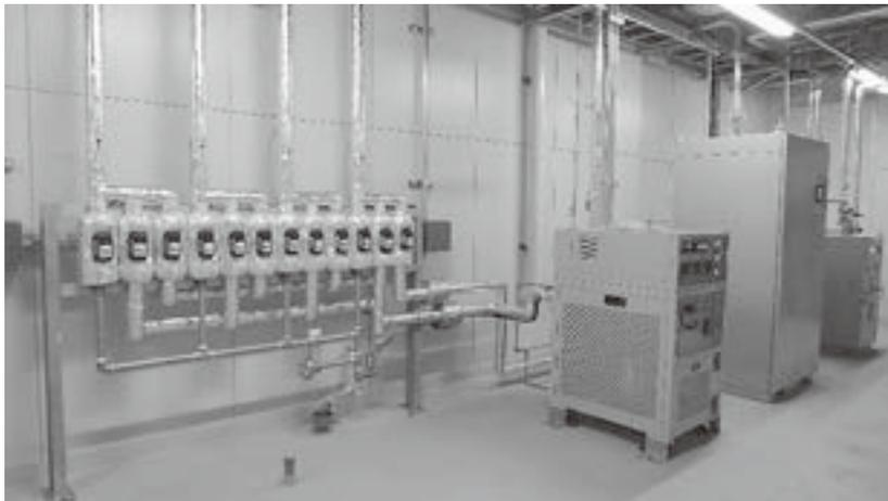
**Photo 6** Machinery room with a nitrogen generator and a temperature/RH control system (② in Figure 2) (Image by the author, February 14, 2014)
