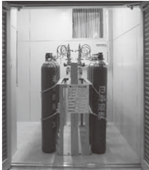
Photo 5 Stock room for carbon dioxide cylinders (① in Figure 2) (Image by the author, February 14, 2014)
