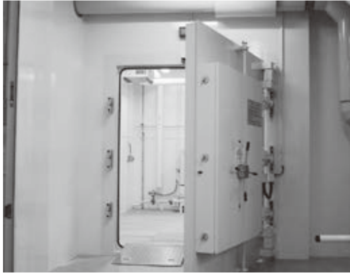
Photo 1 Multi-function fumigation chamber (Image by the author, July 13, 2007)
