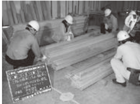
Inspecting before construction
