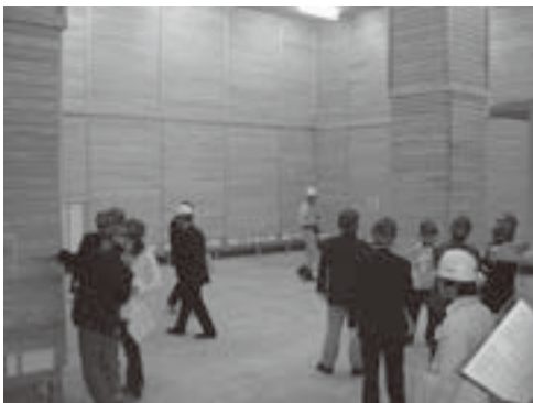
Inspecting during construction
