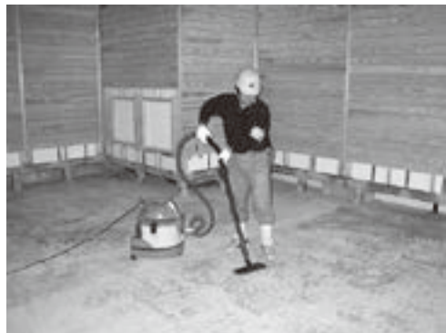
Cleaning after each construction stage
