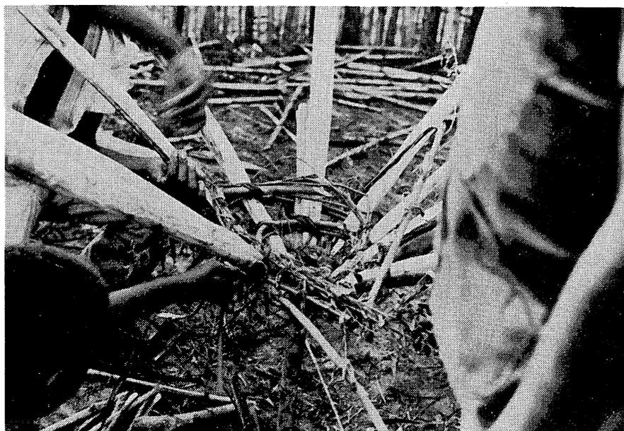
Photo. 2. A ring of withered banana leaves (*ngatta*) is tied horizontally to the top of the *kashonge* and pointed ends of rafters radiate from the *ngatta*.
